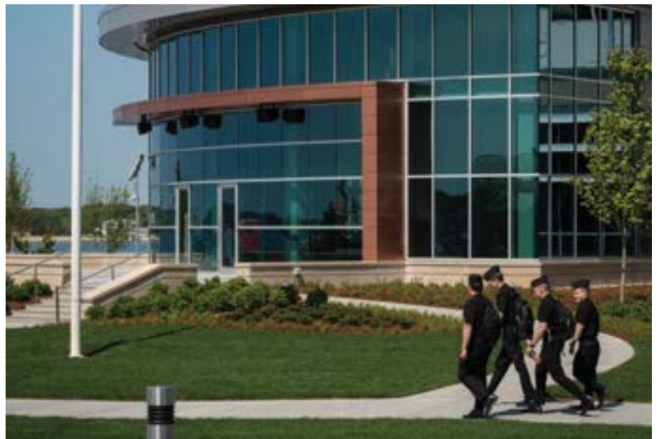
Mess Deck Expansion at Mass Maritime
