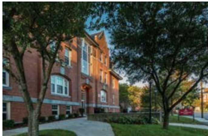
Woodward Hall at Bridgewater State University
