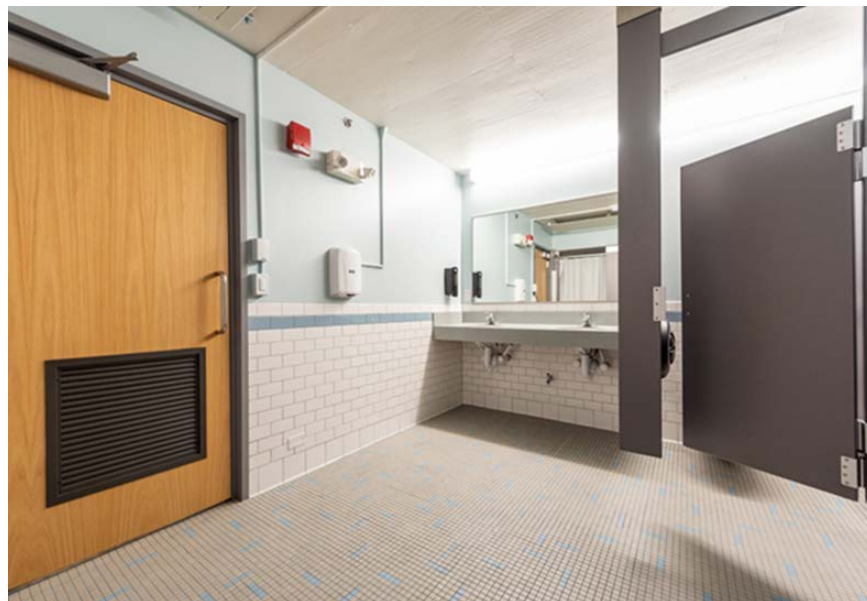
RUSSELL TOWERS BATHROOM RENOVATIONS FITCHBURG STATE UNIVERSITY
