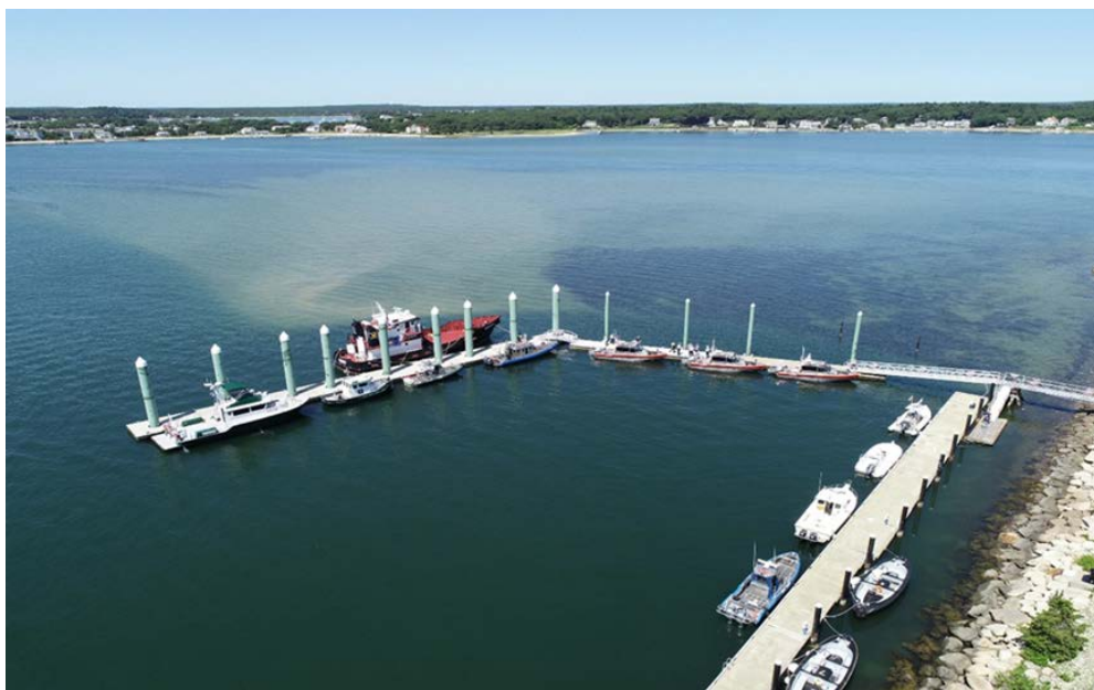
MARINE DOCK RENOVATIONS MASSACHUSETTS MARITIME ACADEMY
